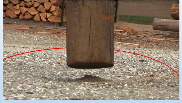
This task is to raise the pole from horizontal (starting on the ground) to near vertical, all the while keeping the pole butt inside the 6 ft. circle. Task is complete when the butt just comes up clear of the ground.
